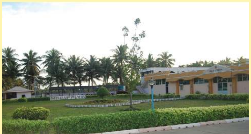
Haripriya Marine Export Pvt Ltd facilities near Bhimavaram town
